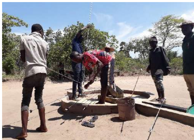
Repair of a structure by a village committee (Mogincual district)
