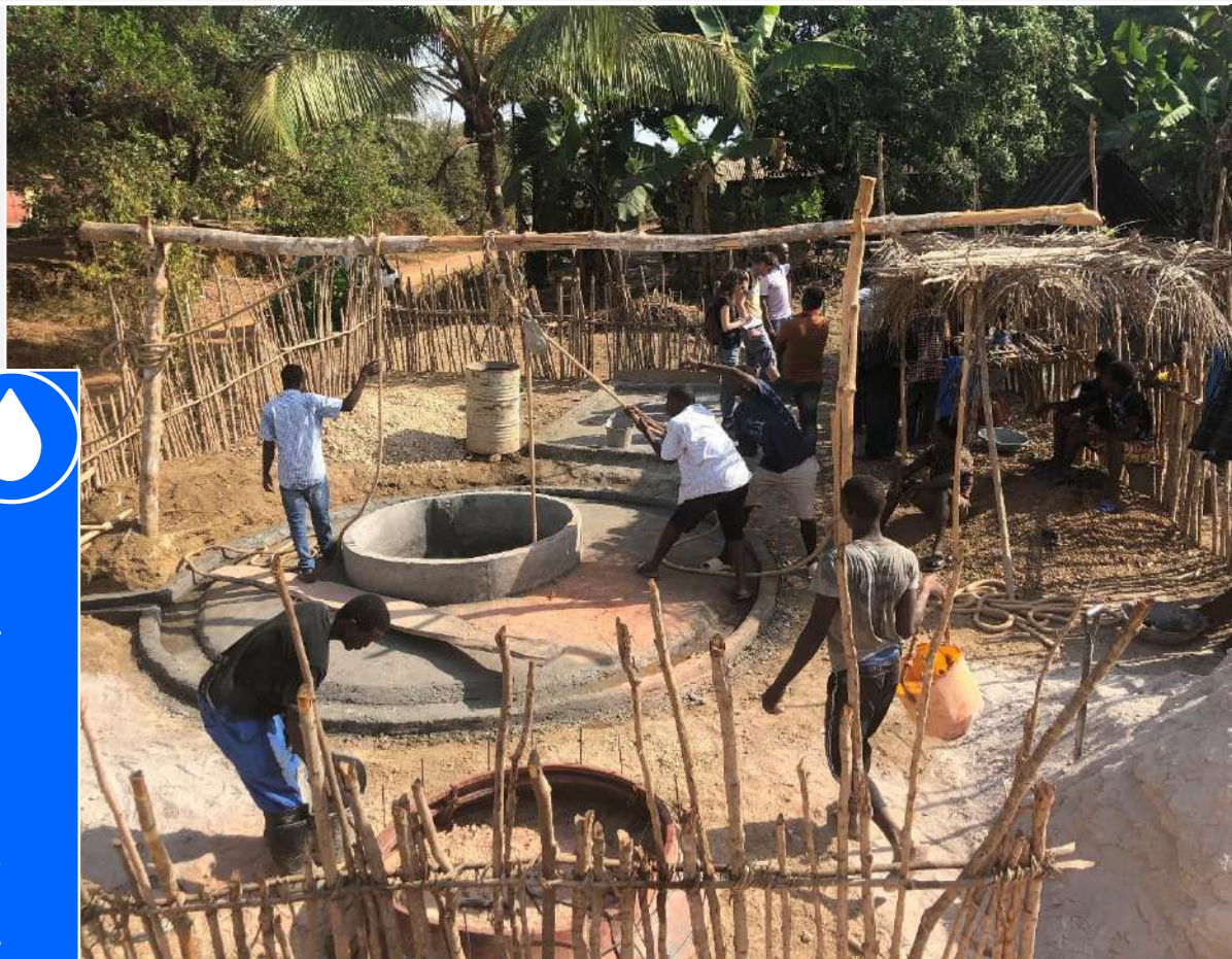
Co-construction of a protected well, Sierra Leone
