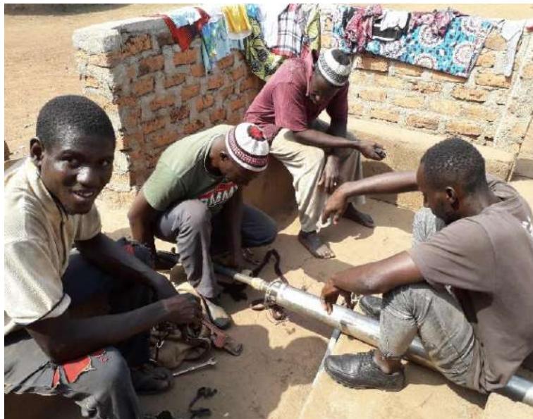
Repairs by the Koumban craftsman (Vergnet pump)
