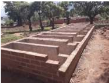
Construction of latrines with pits in a primary school in Phalombe
