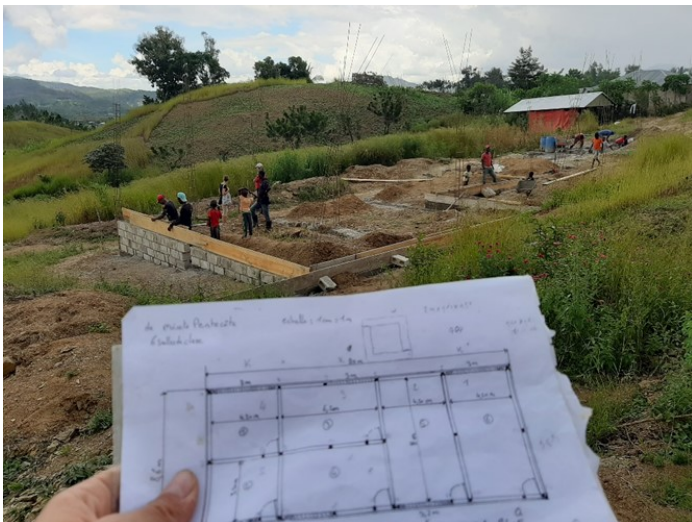
Ongoing construction of a mixed school in Pentecôte de Tilory — Lamielle. The work plan has been adapted to go from 4 to 6 classrooms.
