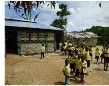
The school of Zabriko have now two buildings to receive children
