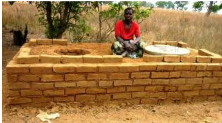
Left : raised lining recently completed. Above : raised lining with compacted soil and slab.
