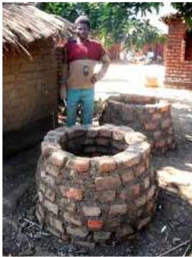
Left : raised lining recently completed. Above : raised lining with compacted soil and slab.
