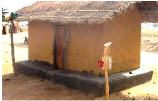
Above : good quality of the superstructure. This Fossa-Alterna is slightly raised.
