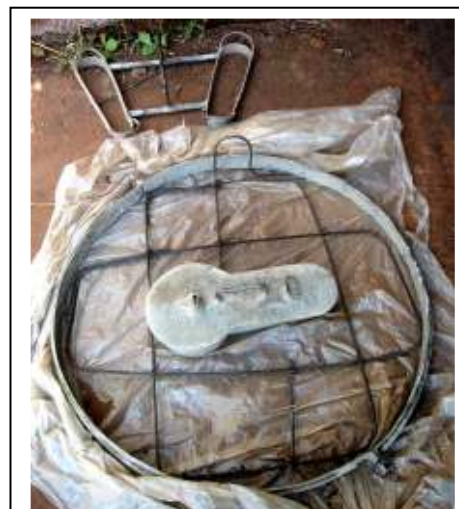
Above: finalized iron frame and moulds just before casting.
