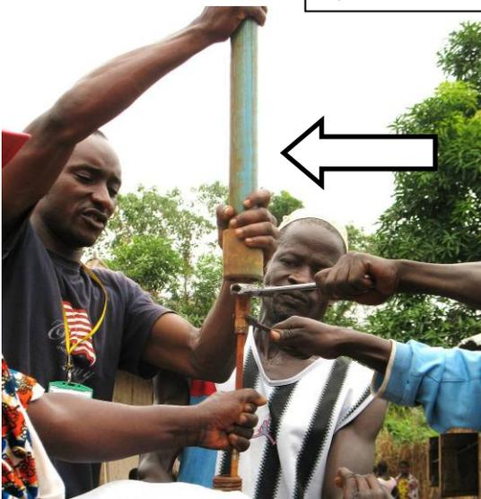
2) During the disconnection of the rod, make sure that someone hold the upper riser pipe section and upper rod vertically
