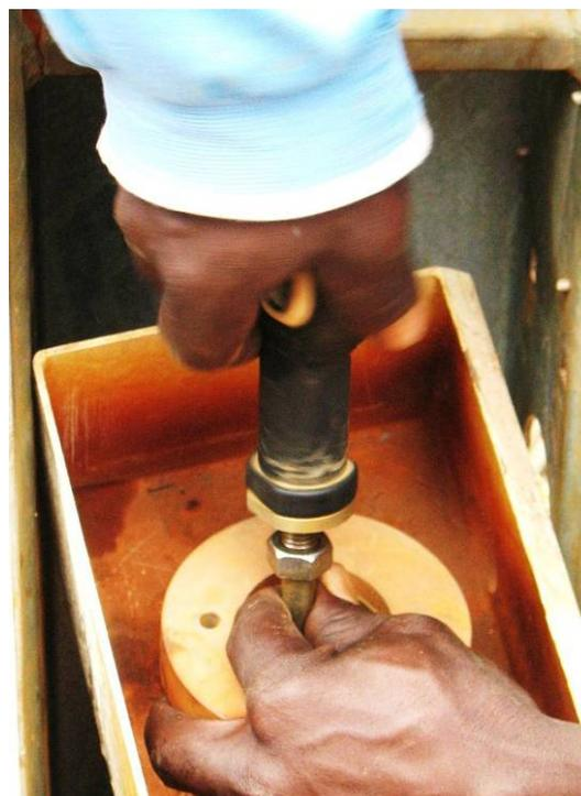
Once the hand lever is disconnected from the linkhead, unscrew the linkhead from the rod
