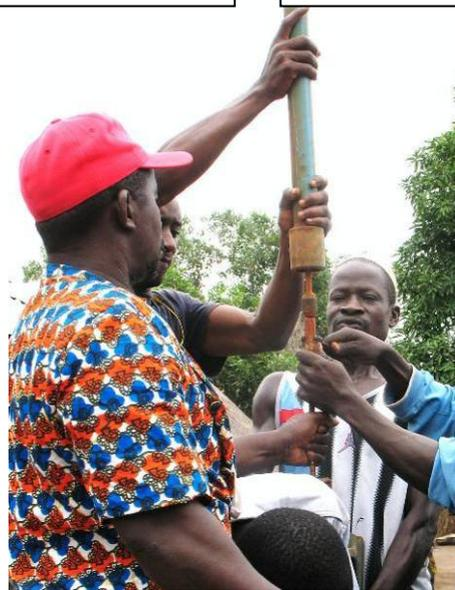
4) Screw riser pipe into double socket. Be careful not to damage the threads. Therefore, always hold riser pipe vertically. Screw slowly into double socket. Connect hand tight only
