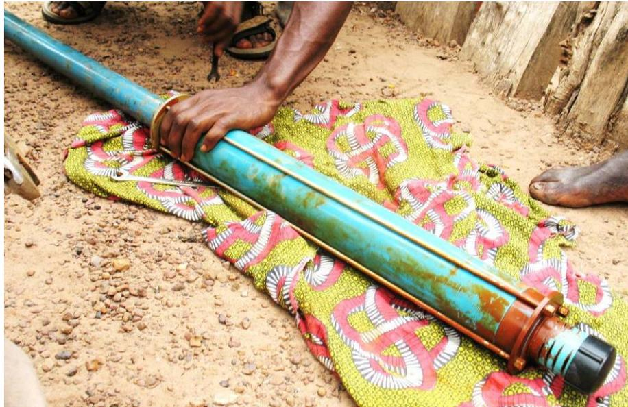
1) Once the last riser pipe section and rod is dismantled. Lay down the cylinder of the pump unit. Keep it away from sand and dust.
